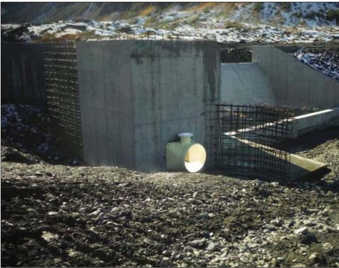
The Allison Creek Hydroelectric Project wrapped up its second construction season in October. This year's work plan focused around the building of the diversion structure, the installation of the penstock, and the inside work at the powerhouse.
