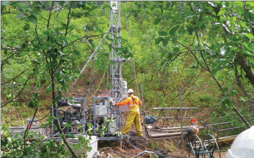
**Left, contractor crews performing boring tests to help determine the geological conditions of the project site**
